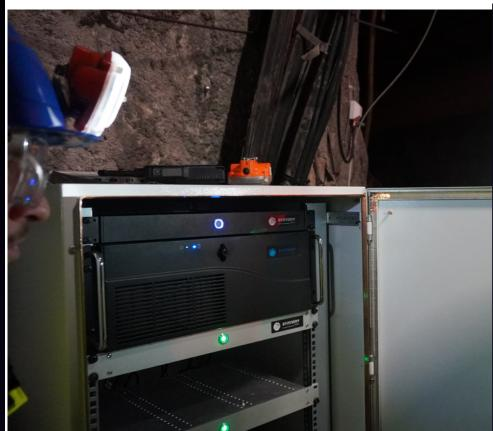
SubWAVE™ is a real-time GPS\* emulator providing signal in facilities out-of-range from natural GPS.
